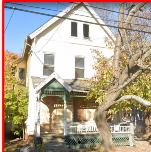
287 Division St Vacant home
