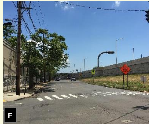
Water St at Olive St (facing west)
