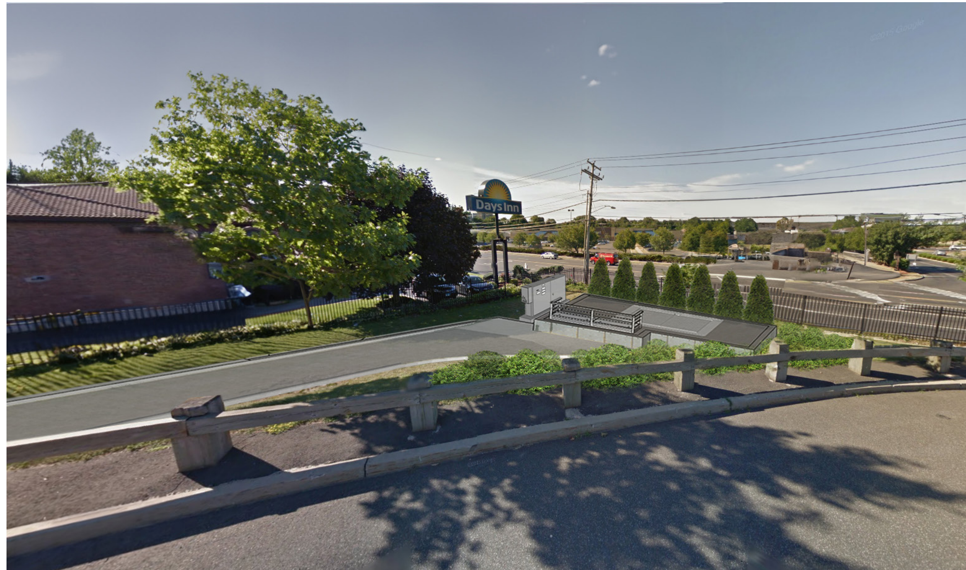
VIEW 1 - FROM SCHOOL DRIVEWAY LOOKING SOUTH
