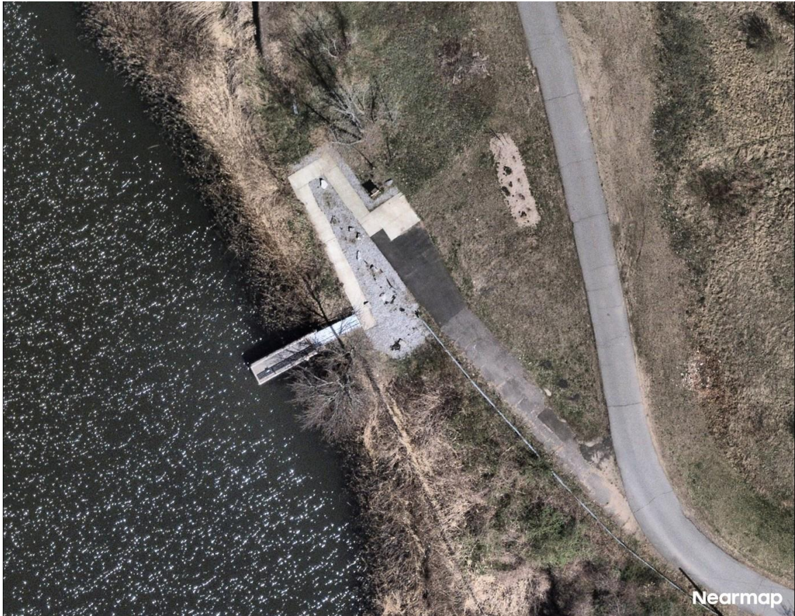
Location at North Pond of Beaver Ponds Park where the new pier will go to replace the current pier.
